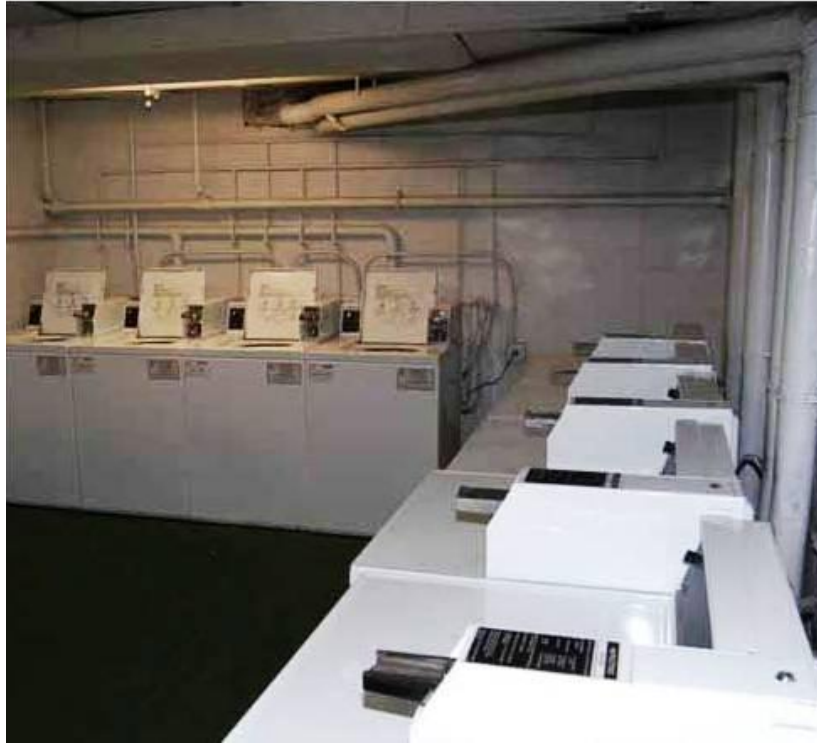
Pre-Renovation: Laundry facility located in the basement
